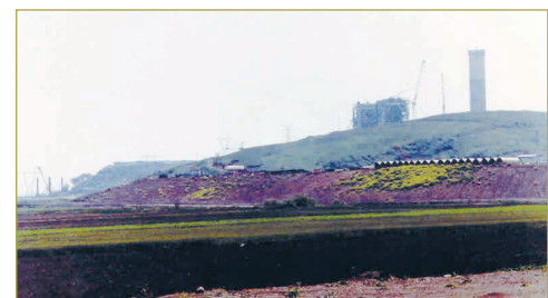
Sugozu Power Plant
