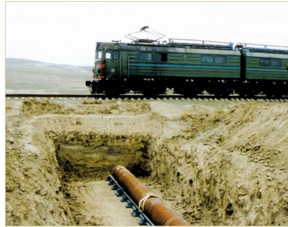
Pipeline passing beneath railway line
