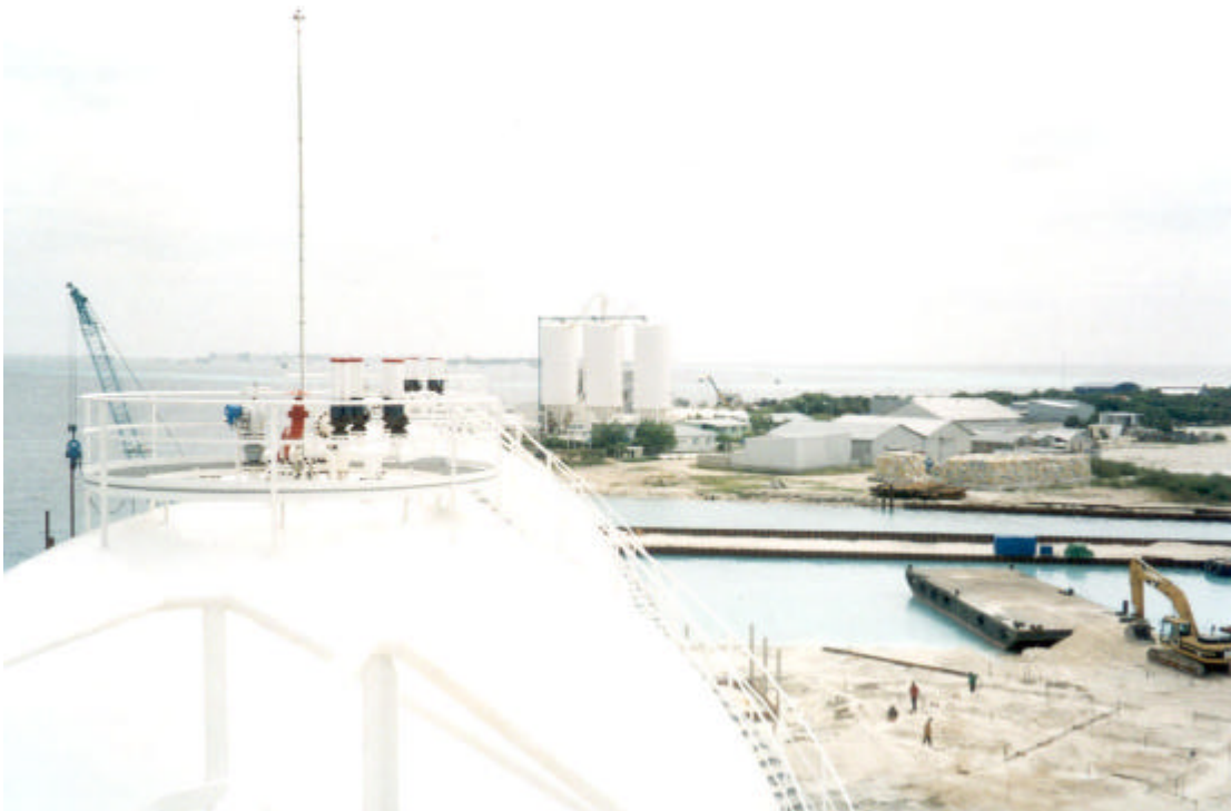
Bulk cement terminal and LPG storage and bottling plant of STO
