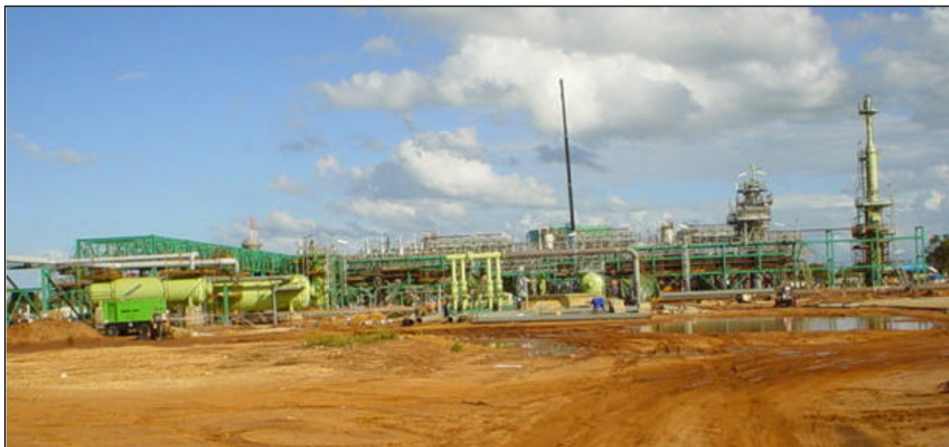
Photograph 5: The Central Processing Facility under construction
