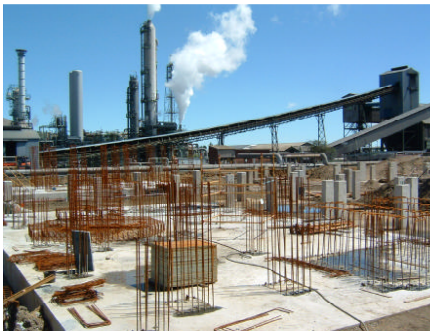
Photograph 11: Foundation of the Reformer in Progress at the Sasolburg plant
