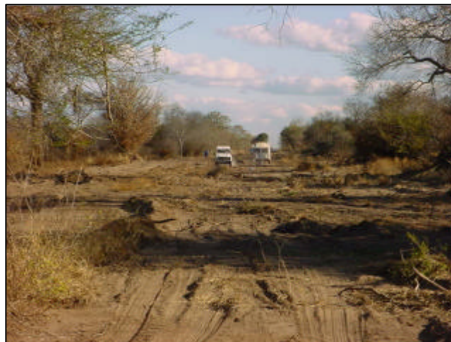
Photograph 15: The pipeline right-of-way in Mozambique
