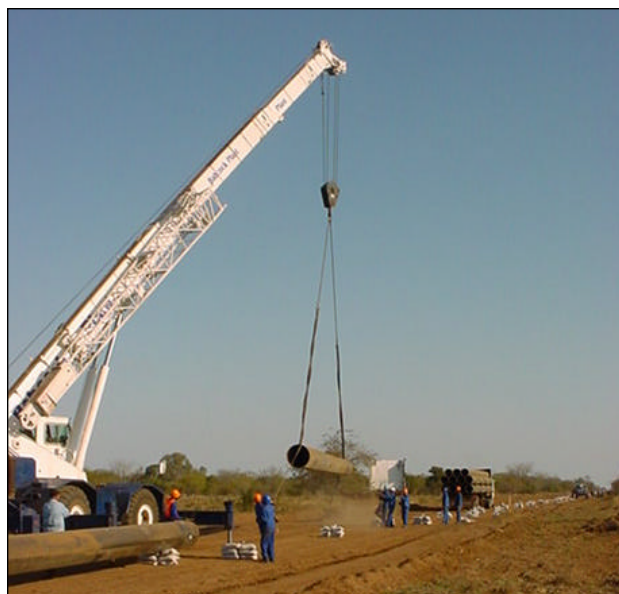
Photograph 6: Stringing of the Pipe along the right-of-way in Mozambique
