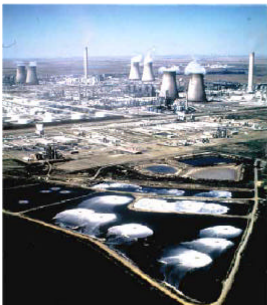
Photograph 10: Sasol Secunda Plant
