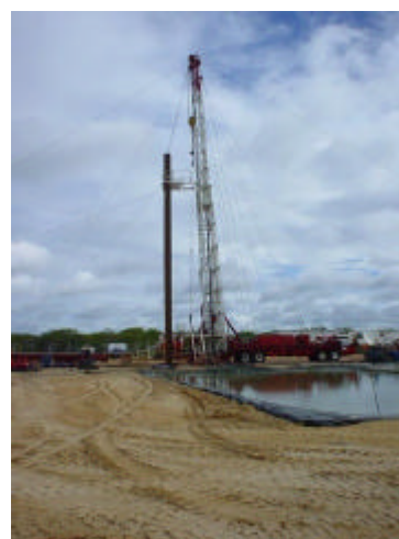
Photograph 3: Drilling rig exploring gas reserves in the Temane Gas Field area: Mozambique
