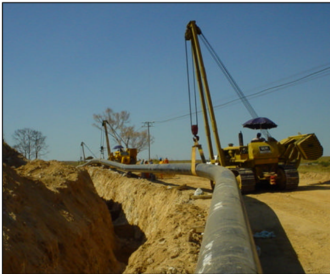
Photograph 9: Laying of the pipe between Komatipoort and Secunda: South Africa
