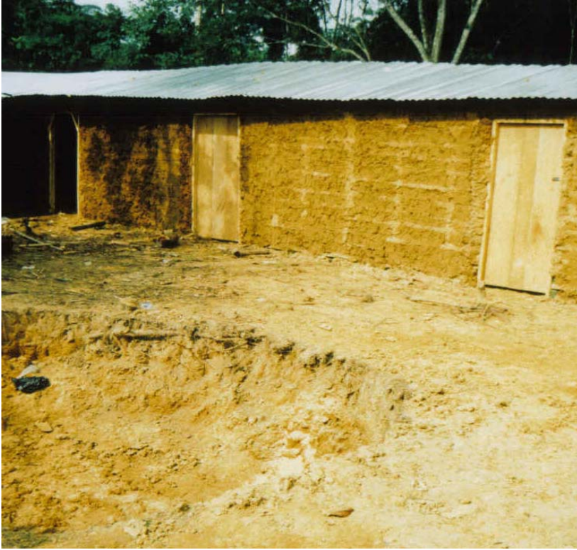
Plate 5: New structures being erected within the affected area.
