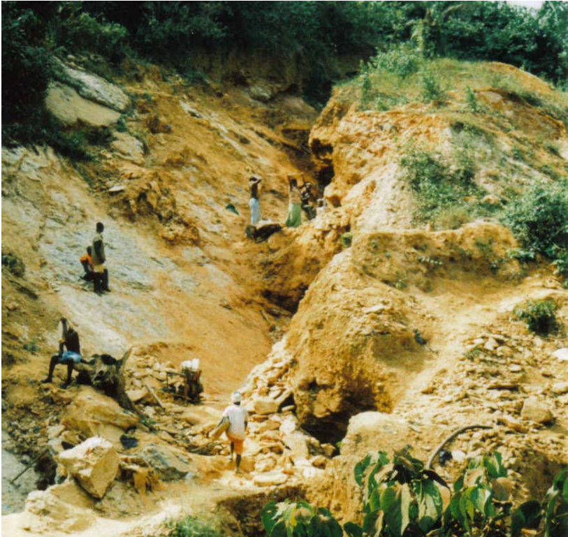
Plate 6: Galamsey operations along the main road leading into Tarkwa.
