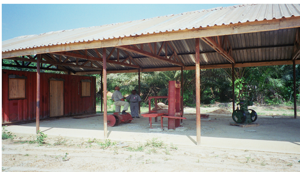
Photo 3-4 Potential palm oil processing shed near Mile 8
