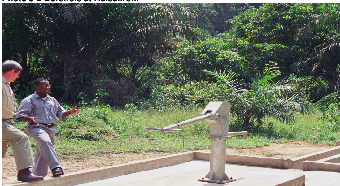
Photo 3-2 Borehole at Adisakrom
