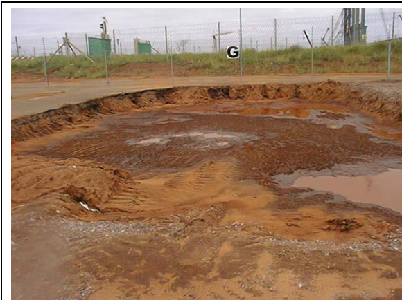
Figure 2: The site under rehabilitation.
