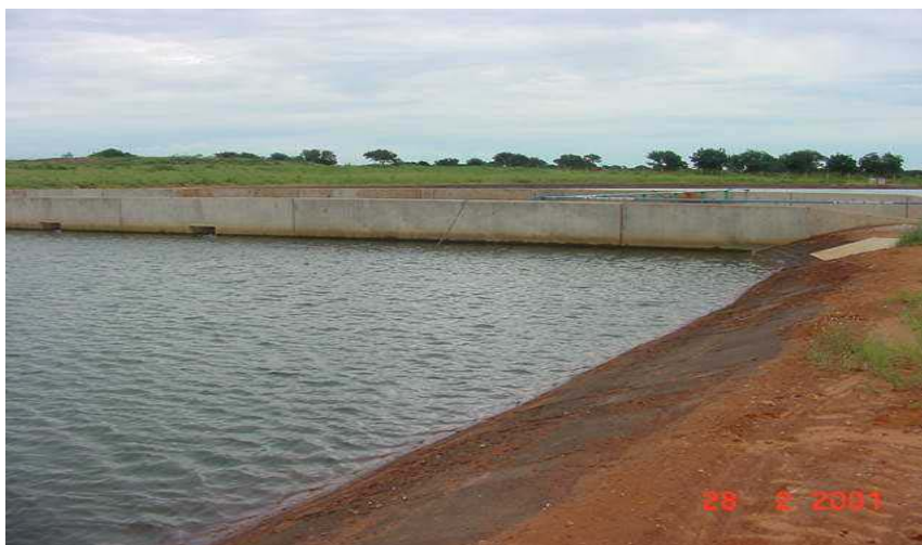
Figure 6: View of the south dam, one of two that provide for the impoundment of stormwater containing fluoride from the smelter site. The complete dam can be seen in the cover photo of the entire smelter site.
