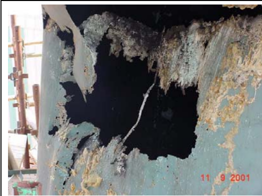
Figure 2: The corroded area of the Cooling Tower.
