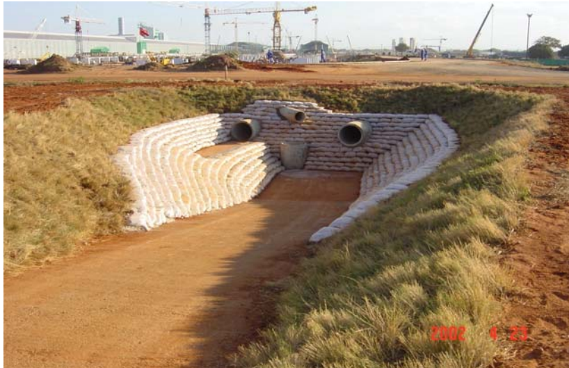
Figure 16: Photograph showing secondary sediment traps on construction site.
