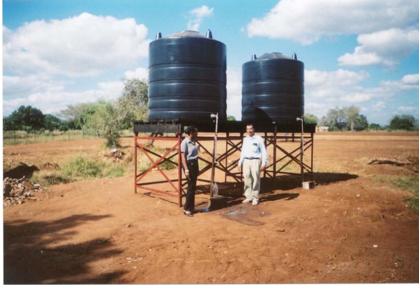
Figure 20: Photograph showing drinking water provision in rural areas.
