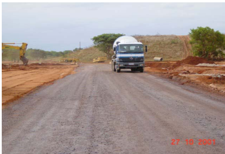
Figure 15: Photograph showing construction road treated with dust suppression palliatives.
