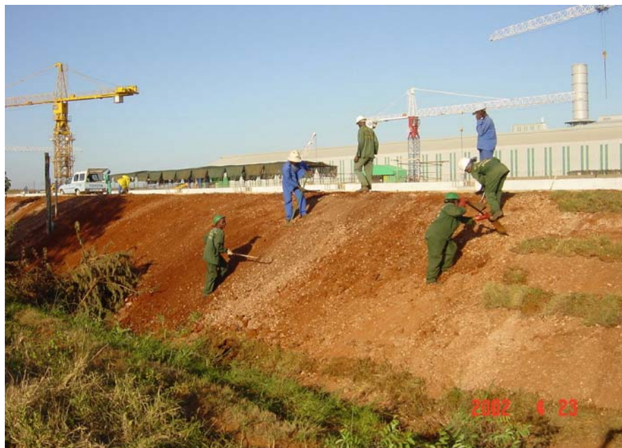
Figure 17: Photograph showing stabilisation of water channels and road embankments with grass
