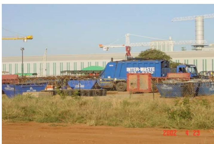
Figure 18: Photograph showing the waste transition station established during the Aluminium Expansion Project to provide for the segregation and safe disposal of waste generated during the project.
