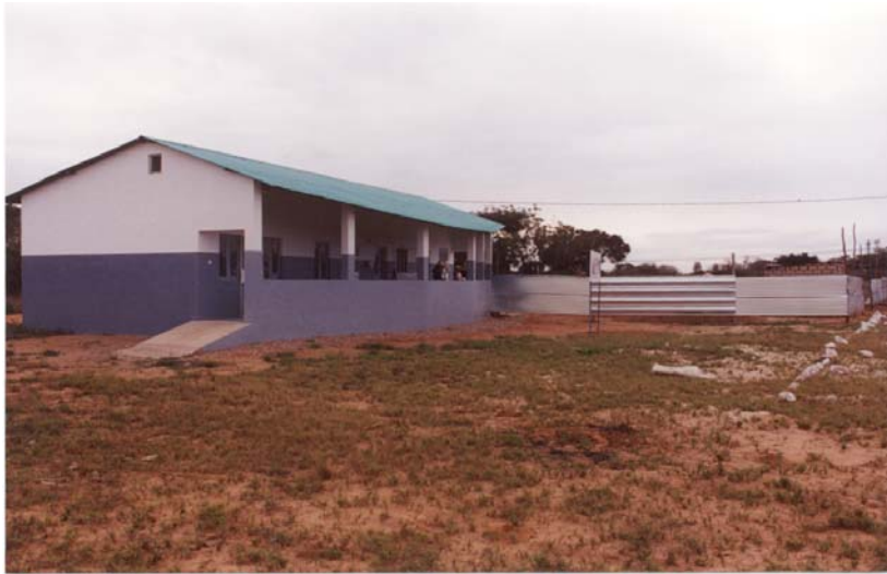
Figure 24: Photograph showing the Beluluane maternity child health care centre.
